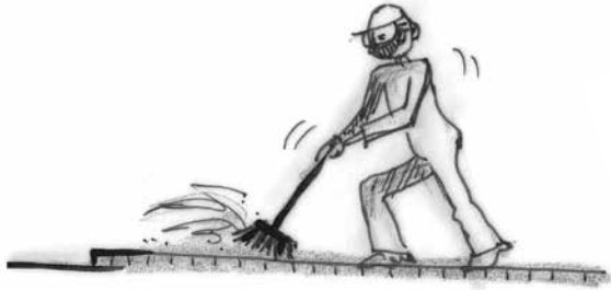
Sweep all debris from pavers before compaction
