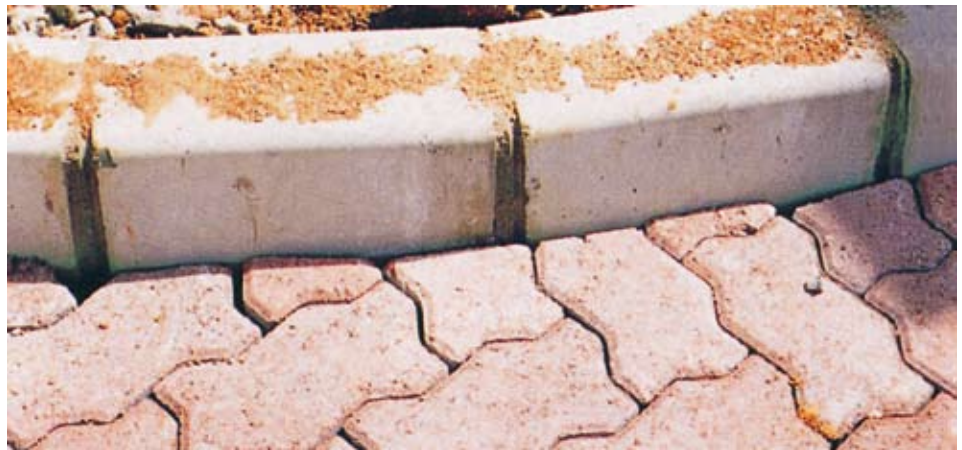
Cutting blocks at edge restraints
