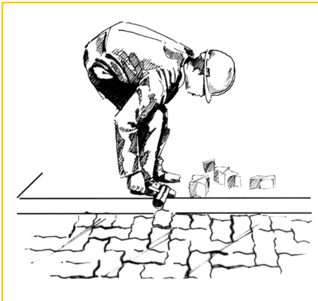
Figure 13: Fitting cut blocks into gaps
