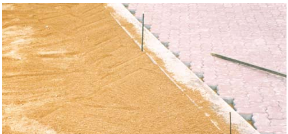
Temporary restraint at end of a days production
