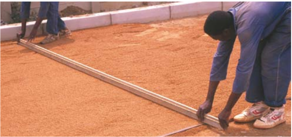
Screeding the bedding sand
