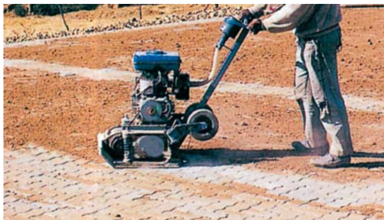
Vibrating the jointing sand into the joints
