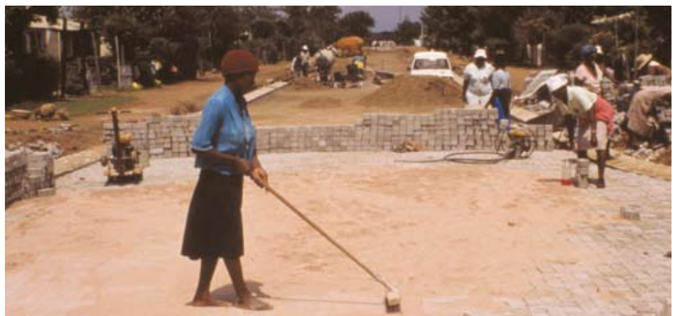
Sweeping in the jointing sand
