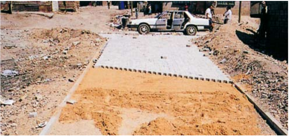
Typical site layout/ construction sequence
