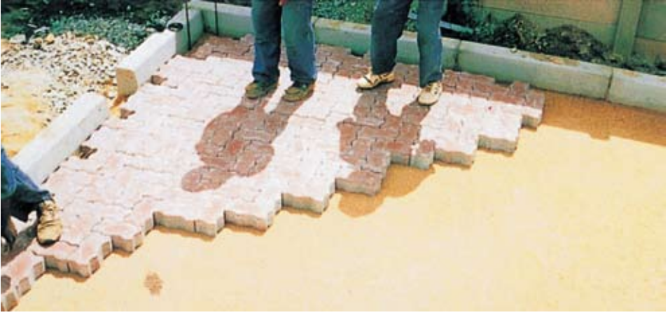
Commencement of laying establishing a diagonal face
