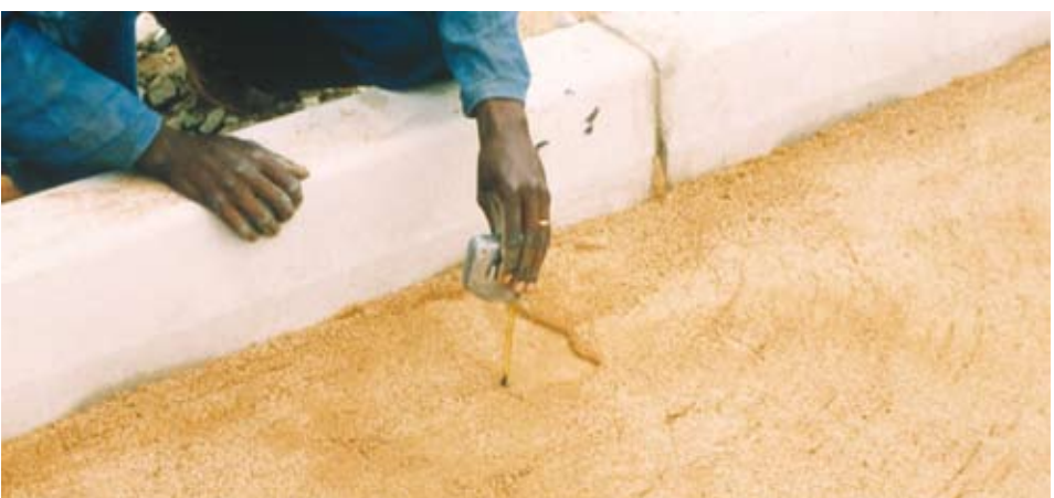
Edge restraints installed before laying commences
